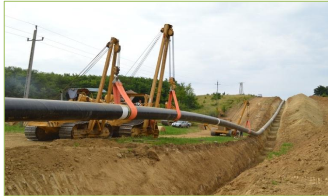
Some parts under construction
