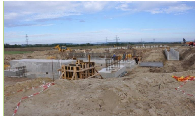
Compressor station at Szada
