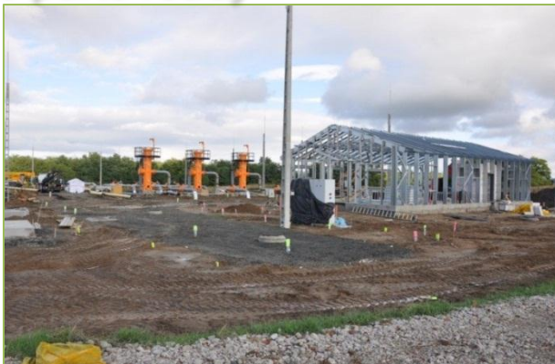
International metering station at Balassagyarmat
